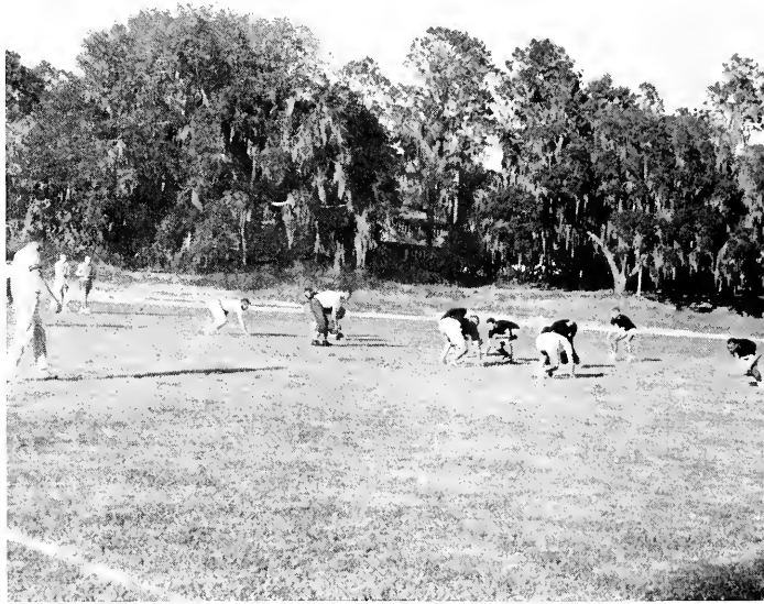
Ready for the snap down on the new athletic field.
