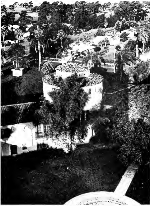
The Granary Tower
