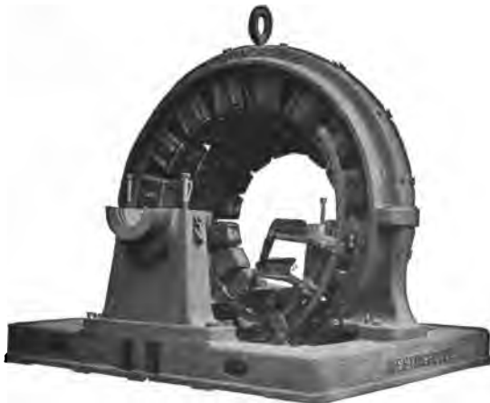
FIG. 2,065.—Westinghouse field frames and bearings for synchronous booster rotary converter. The frames consist of heavy cast yokes. The poles are fastened to the frames with through bolts. The bed plate is in one piece for the small machines and in two pieces for the large ones.
