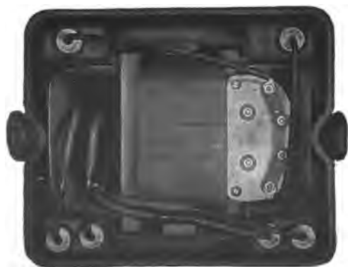
FIG. 1,943.—Top view of Fort Wayne (type A) transformer cover removed, showing assembly of coils and core and disposition of leads.
