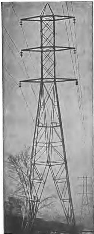
FIG. 2,190.—General Electric standard tower for high tension three phase transmission line.
