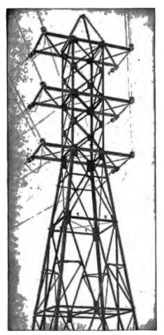
Fig. 2.148.—Angle tower showing General Electric strain insulators. The tower being subject to great tortional strains is creeted on a massive concrete foundation. The construction is similar to the standard tower but of heavier material, and having the same vertical dimensions but with bases 201t. aquare.
