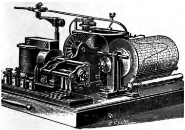
5. 2,598.—View of Hospitalier ondograph. In operation, a long pivoted pointer carrying a pen and actuated by electromagnets, records on a revolving drum a wave form representing the alternating current, pressure or current wave.
