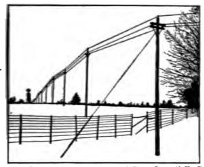
4.—View of a three phase, 2.300 volt, 60 cycle line at Charr, N. Y. The current is smitted at the alternator voltage 23, miles over the single circuit pole line. The rare of cedar with fir cross arms, and are fitted with pin insulators. They are from 5.40 feet high and are spaced at an average of about 120 feet. The conductors are copper wire No. 00 B. & S. The alternators consist of one 50 kw., and one 100 kw. rral Electric machines.
