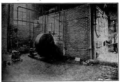
2747.—Forced draft plant with hollow bridge wall at the Crystal Water Co., Buffalo-N. Y. The air is delivered to the ash pit via the hollow bridge wall, being supplied under pressure by the blower seen at the side of the boiler setting. As shown, the blower is operated by a small reciprocating engine; however, compact blowing units with steam turbine drive can be had and which are designed to be placed in the boiler setting.
