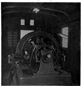
Pig. 2,780.—Westinghouse 300 kw. converter in portable sub-station.
