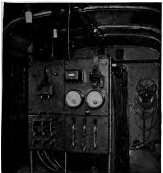
© 2,781.—Switchboard end of Westinghouse portable sub-station.
