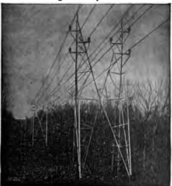
2.189.—Twin circuit "aermotor" towers carrying 44,000 volt conductors (Southern Power Co.). These towers vary in height from 35 to 50 feet, and the circuits are transposed every 10 miles. The towers are assembled on the ground and erected by means of gin poles. They are normally spaced 500 feet apart with a sag of 5 feet 8 inches. The minimum distance between towers is 300 feet and the maximum 700 feet.
