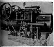
2.772.—Buckeye mobile, or self contained unit consisting of compound condensing encues, boller, superheater, reheater, feed and air numps; it produces one horse power on 1½ lbs.
