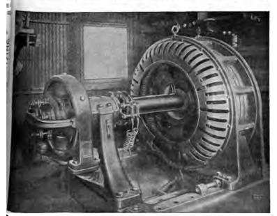
2479.—General Electric 400 kw., 550 volt, 600 R.P.M., synchronous condenser with direct connected exciter installed in sub-station No. 1 of the Colorado Light & Power Co., Cripple Creek, Colo. The machine is designed for alternating current starting by means of a compensator. The field is provided with a standard synchronous motor winding, and, in addition, an amortisseur winding which assists in starting and serves as a damping device to minimize hunting.
