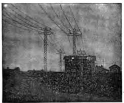
Pig. 2.138.—44,000 volt lines entering the Gastonia sub-station of the Southern Power Co. The poles used are of the twin circuit two arm type, built of structural steel, their height varying from 45 to 80 feet, the latter weighing 9,000 pounds each. These poles have their bases weighted with concrete.
