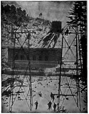
Fig. 2,173.—Beginning of Schaghticoke-Schenectady transmission line; view showing towers with power house in background.
