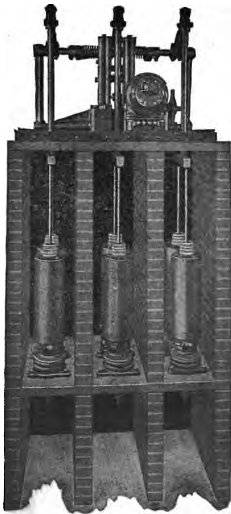
FIG. 2,232 —General Electric motor operated three phase oil switch. The operation of the oil switch is accomplished by a small hand controlling switch, generally mounted on the panel, with the instruments which are in the circuit controlled by the oil switch. The standard pressure for the operating motor is 125 volts. The switch has six breaks, each break being in a separate tank. In addition to this isolation of the breaks, each phase is enclosed in a fireproof brick compartment, making it impossible for trouble in one phase to be communicated to another. The cells are constructed of brick with top and bottom slabs of slate. The capacities of such switches, range from 2,500 to 60,000 volts, and from 100 to 1,000 amperes.
