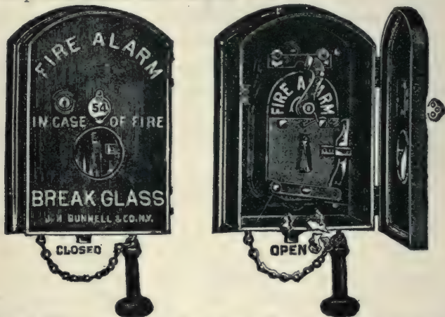
FIGS. 3,317 and 3,318.—Jupiter fire alarm box closed and open with glass broken and alarm going in. In operation when glass is broken the mechanism acts automatically, sending in the number of the box four times. Once starting, the alarm cannot be interfered with. By means of a special key the circuit and mechanism may be tested or a single round of the box sent in as a watchman's signal without disturbing the glass or interfering with the regular fire alarm setting of the box. The inner box contains the signal movement. On the front of the inner box is mounted the trip and latch that engages the pull lever of box holding it in set or wound position until released by breaking the glass.
