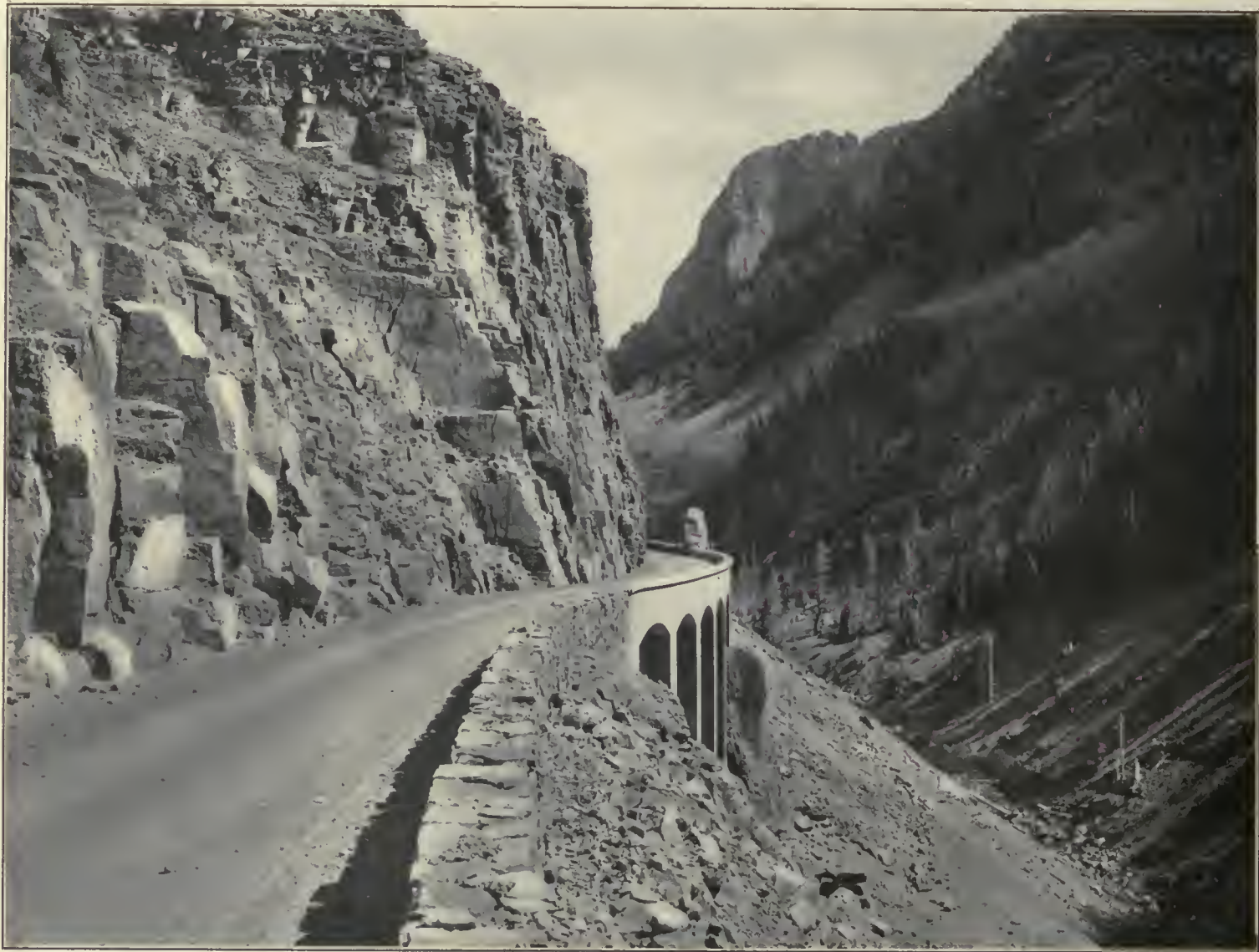
GOLDEN GATE CANYON AND VIADUCT
