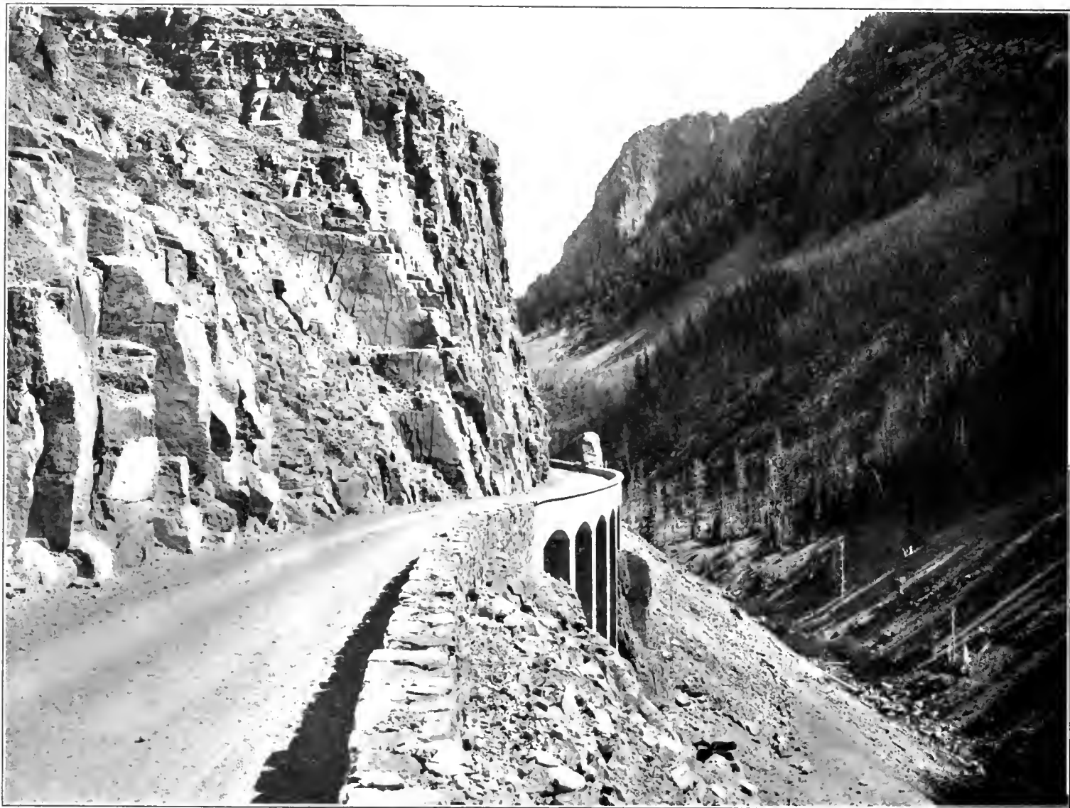
GOLDEN GATE CANYON AND VIADUCT
