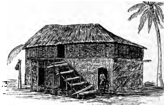
FIG. 20. HOUSE ON PILES AT SAIBAI With the lower portion screened with leaves (1888)
