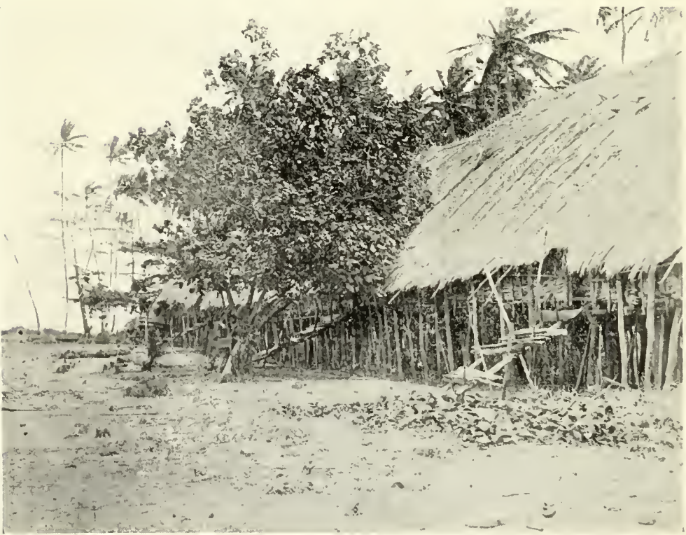
SIDE VIEW OF THE SOKO-KOROBE CLAN HOUSE AT IASA
