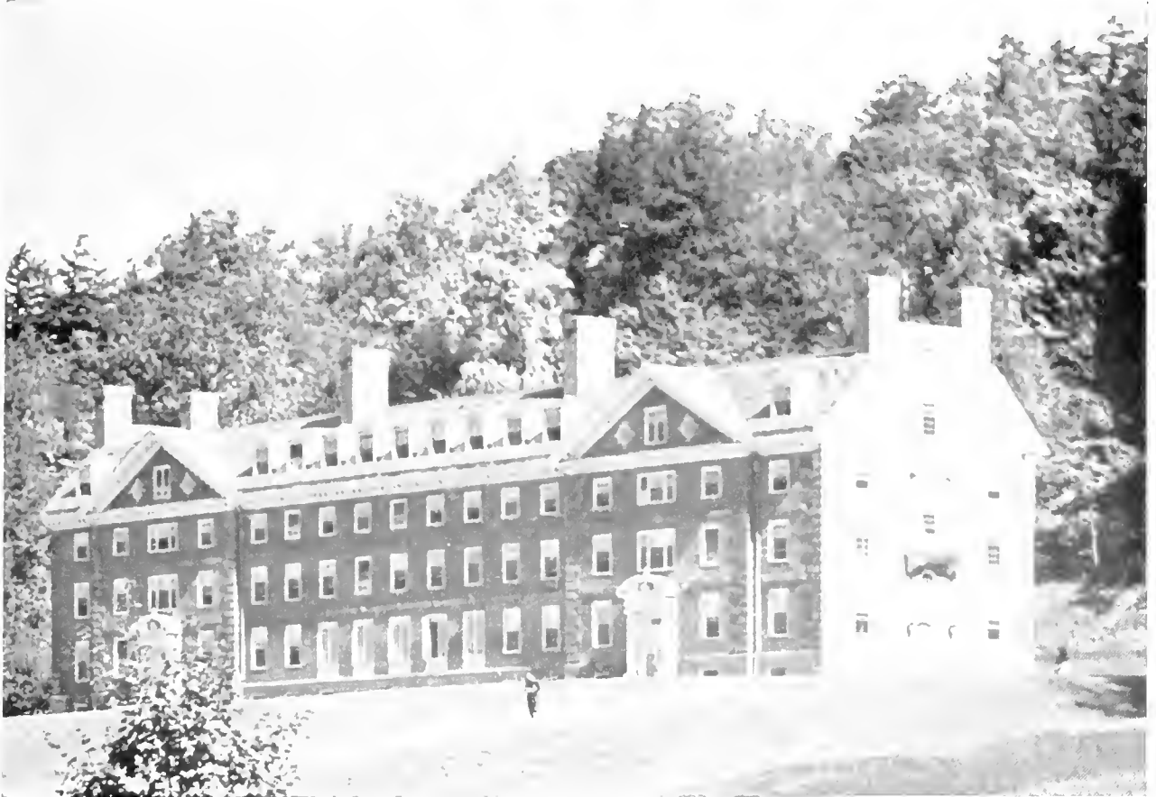
Abigail Adams (top) is Women's Dormitory; Thatcher Hall Houses 150 Men
