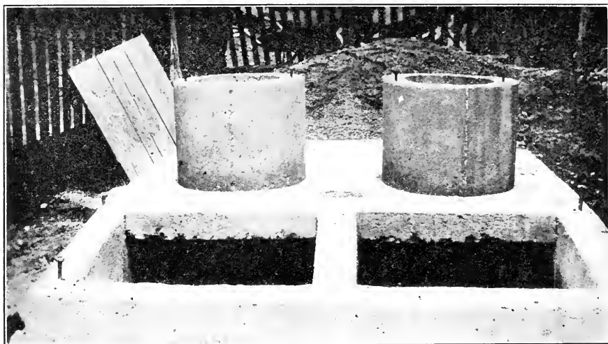
FIG. 21. Double compartment concrete vault, with top and seat risers in position.
