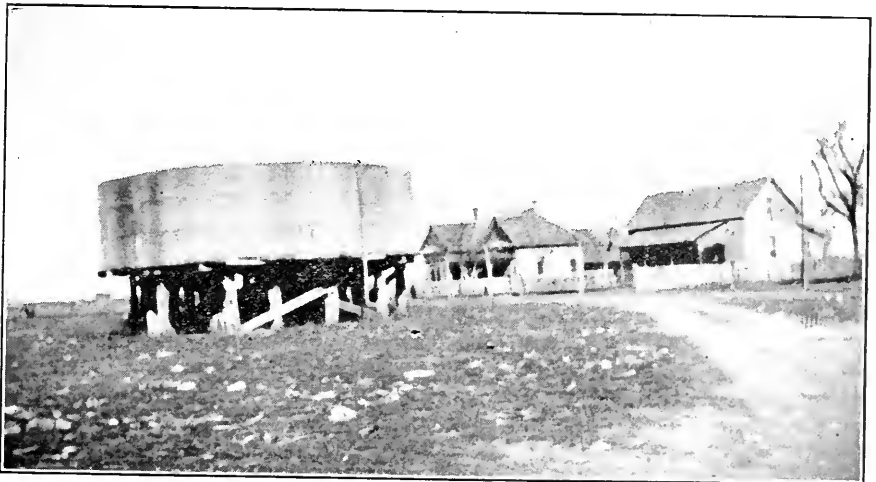
FIG. 4. The effect of winds, etc., on open surface privy filth. Soiled toilet paper was found floating in this tank, having been blown in from the near-by privies.
