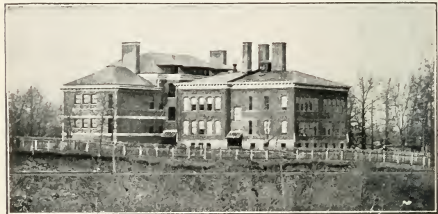
FIG. 3. THREE GENERATIONS OF A SCHOOL BUILDING EAST ORANGE, NEW JERSEY
