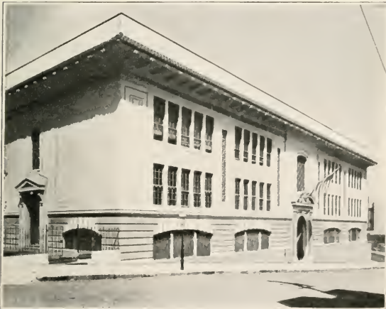
FIG. 2. THREE GENERATIONS OF SCHOOL BUILDINGS SAN FRANCISCO, CALIFORNIA
