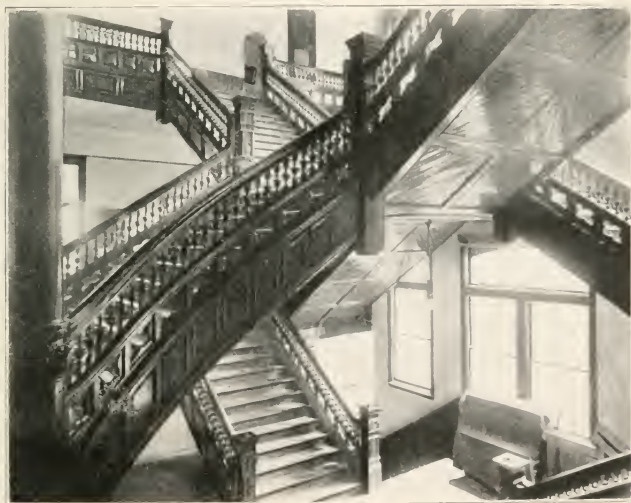
FIG. 18. FIRE DANGERS WHICH NEED ATTENTION
