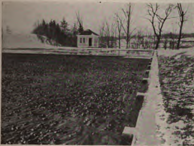
Fig. 50.—Stone bed of a sewage disposal plant.
