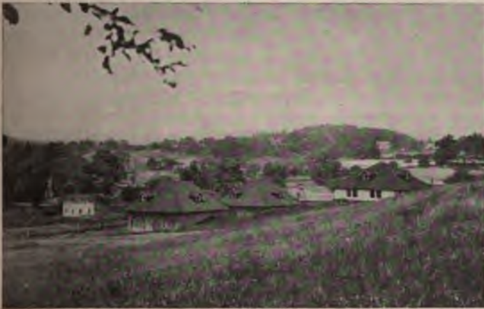
Fig. 51.—View of an attractive sewage disposal plant. The three low houses in the foreground cover the objectionable structures.
