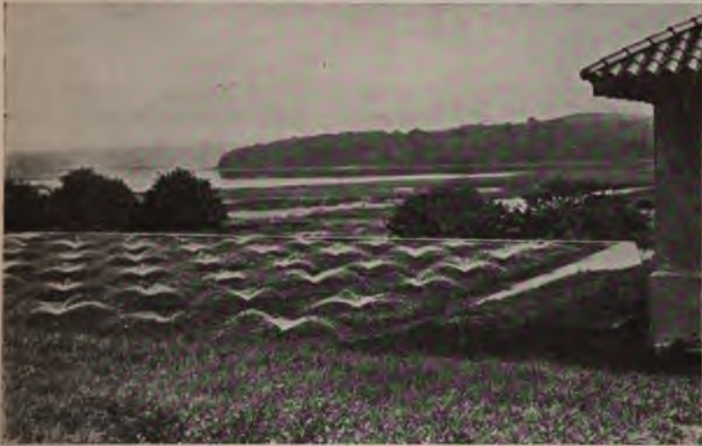
Fig. 46.—Sprinkling sewage over the stone bed of a sewage disposal plant.
