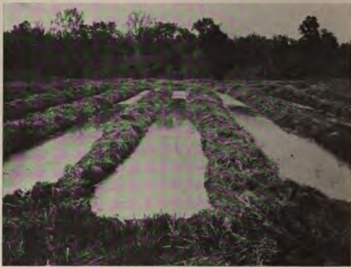
Fig. 42.—Surface disposal of sewage—a crude system.
