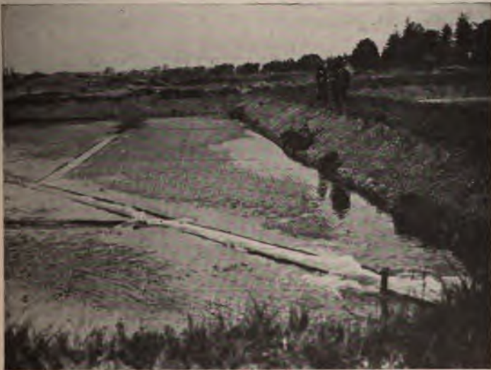
Fig. 47.—Sand filter of a sewage disposal plant.
