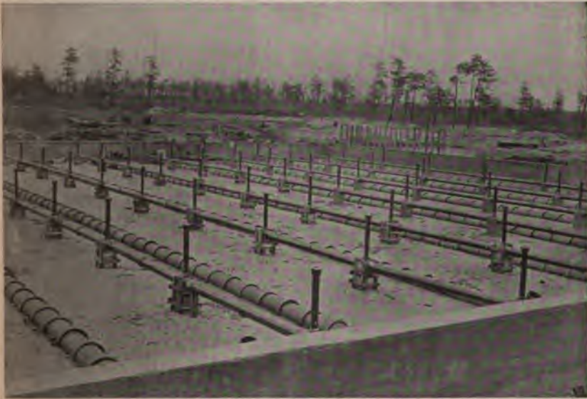
Fig. 44.—The sprinkling pipes and underdraining tiling of the stone bed of a sewage disposal plant ready to be covered with stone.
