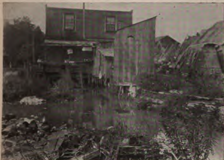
Fig. 41.—Sewage in the interior of a village block that needs a public sewer system.
