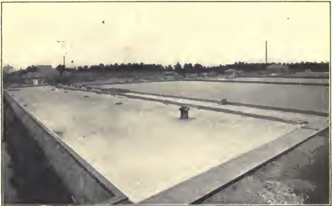
FILTER BEDS OF THE INDIANAPOLIS WATERWORKS.
