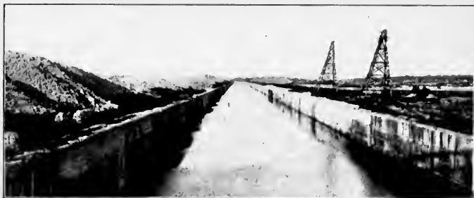
THE CHICAGO DRAINAGE CANAL.
