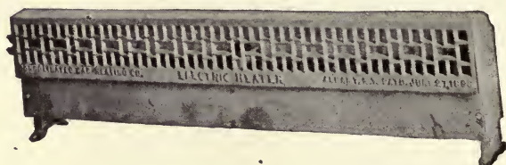
FIG. 276.—Car Heater of Consolidated Co.
