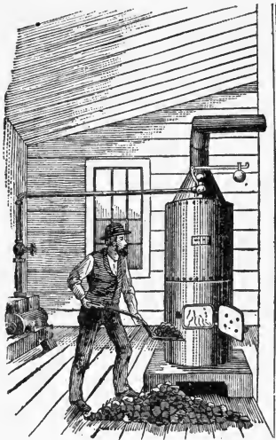
FIG. 186. The Boiler before Explosion.
