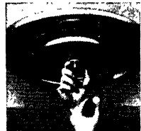
Fig. 6 Air Volume Adjustment
