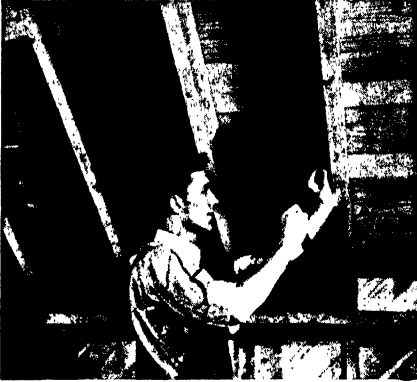
Applying Longfibre Super-Felt batts in new home
