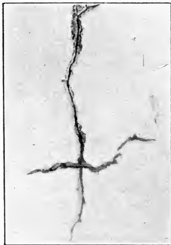
FIG. 45.—Crack in threaded hole of boiler-plate fire-box.
