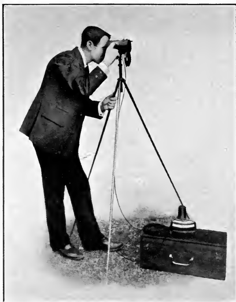
FIG. 56.—Sighting the Féry radiation pyrometer.
