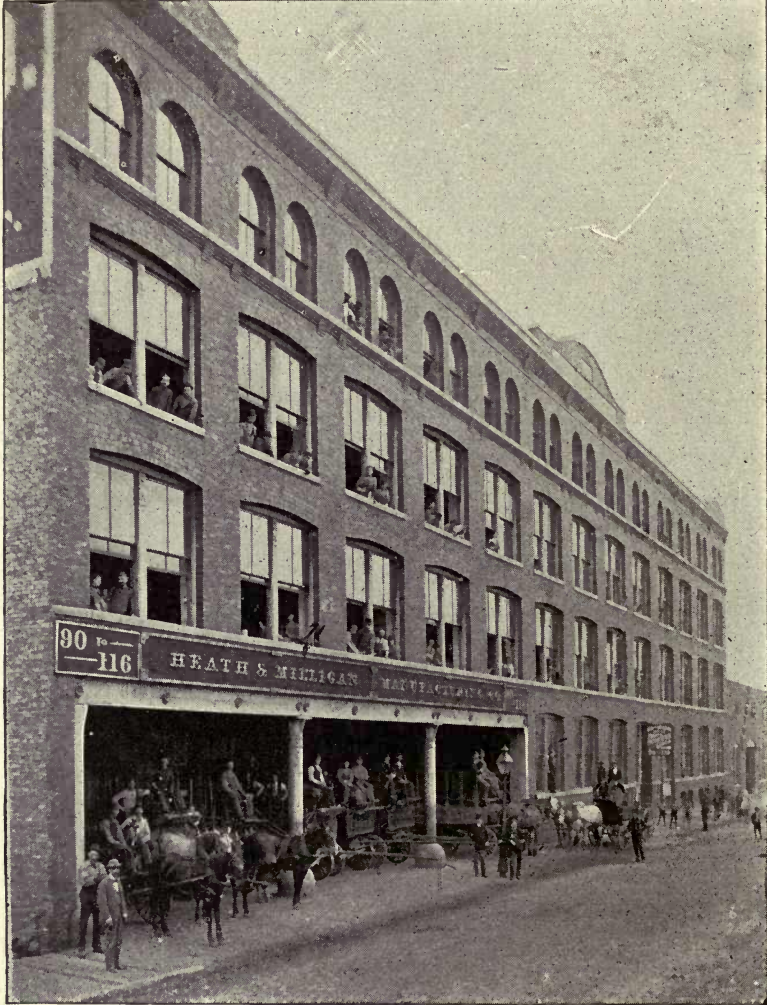
Heath & Milligan Mfg. Co., CHICAGO, ILL. Contains 400 H. P. Heine Boilers.
