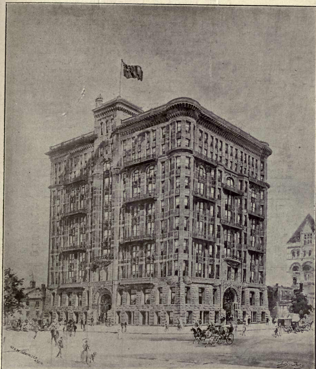
Foresters' Temple. Headquarters of Independent Order of Foresters, TORONTO, ONT., CANADA. Contains 240 H. P. of Heine Boilers.
