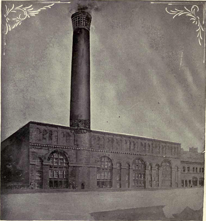
Station C, Edison Light and Power Co., SAN FRANCISCO, CAL. Contains 1500 H. P. Heine Boilers.
