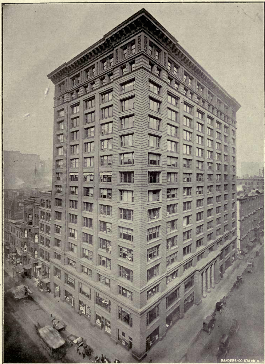
Marquette Building, CHICAGO, ILL. Contains 1000 H. P. of Heine Boilers.
