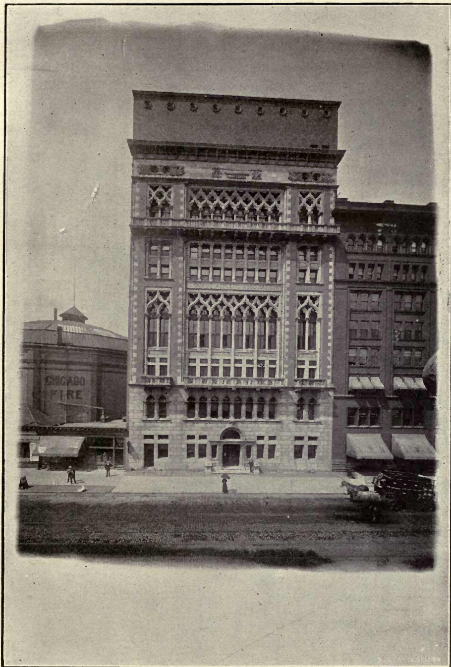
Chicago Athletic Club, CHICAGO, ILL. Contains 300 H. P. Heine Boilers.
