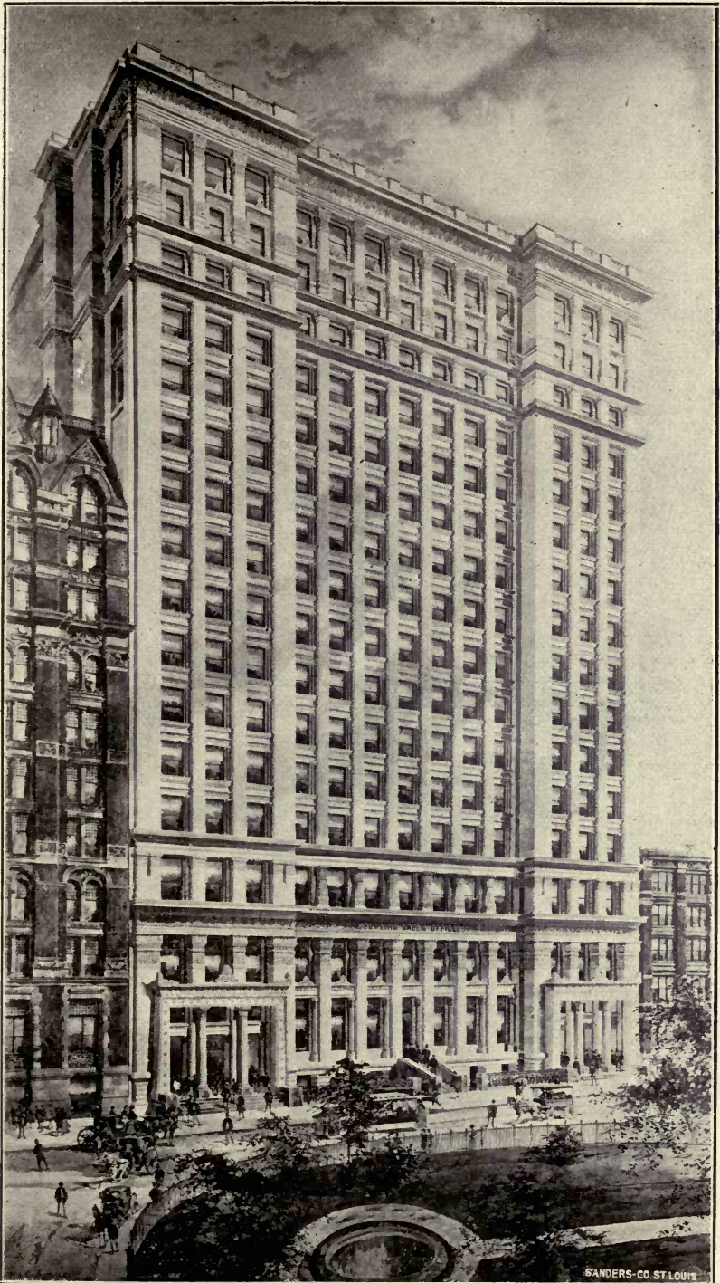
Bowling Green Office Building, NEW YORK. Equipped with 750 H. P. Heine Safety Boilers.
