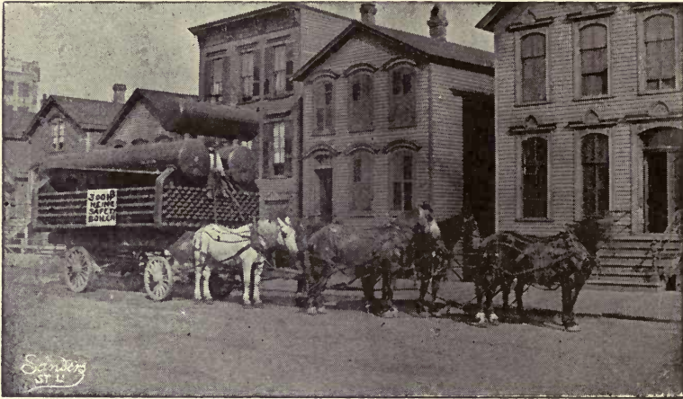
300 H. P. Heine Boiler being moved.
