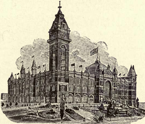
Minneapolis Industrial Exposition Building, Minneapolis, Minn., With Heine Boiler Plant of 1000 H. P.
