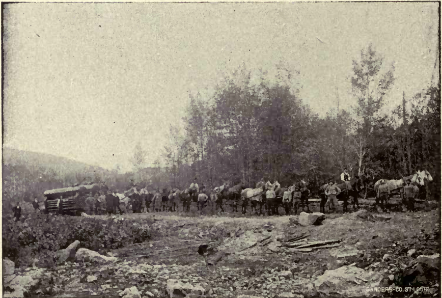
Hauling a 250 H. P. Heine Boiler up a Mountain.
