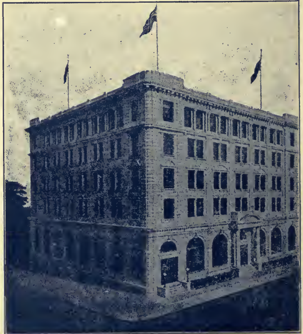
WINCH BUILDING, VANCOUVER
