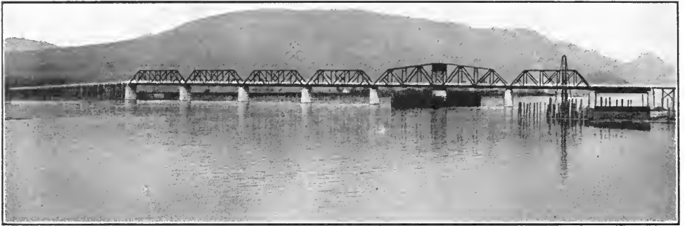
PROVINCIAL GOVERNMENT BRIDGE, PITT RIVER, B.C. Armstrong, Morrison & Co., Ltd., Contractors
