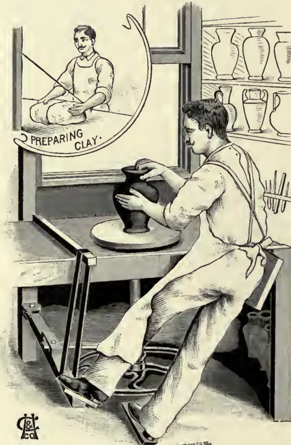
Fig. 5. Shows the modern potter's wheel turned by foot-power.
