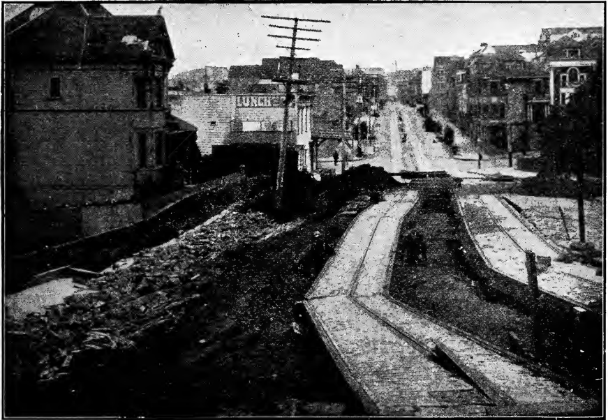
A portion of Union Street, San Francisco, after the earthquake, April 18, 1906.
