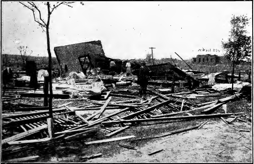
Wreckage in the pathway of the tornado which visited Louisiana, Mississippi, and Alabama, on April 24, 1908. Tornadoes leaving similar destruction in their track during 1908 visited Texas, Oklahoma, Minnesota, Nebraska, Kansas, New Mexico, Iowa, Portugal, and Hungary.
