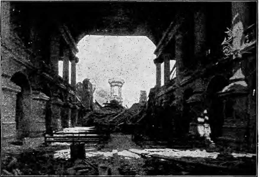
Interior of Merced Temple, Valparaiso, after the earthquake of August 16, 1906.
