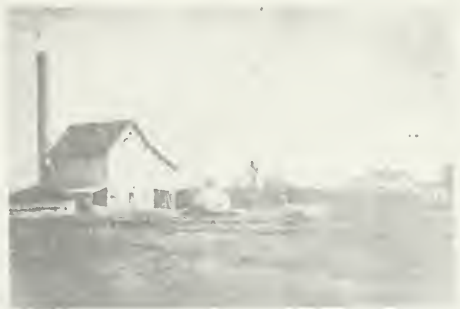
The Barnum Flour Mill was built in 1859 by Hohart and Dickerson. The flour from the mill was called "Empire State".
