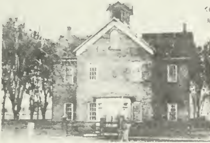
Washington School entrance was on north side.
