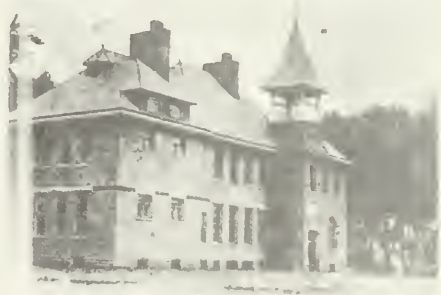
Washington School. New addition was on the south side.
