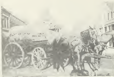
Ed Beckham sprinkles down dust in streets
