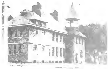
Washington School. New addition was on the south side.
