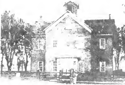
Washington School entrance was on north side.
