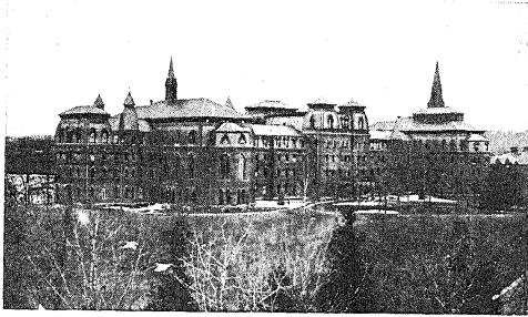
College Hall, destroyed by fire in 1914
