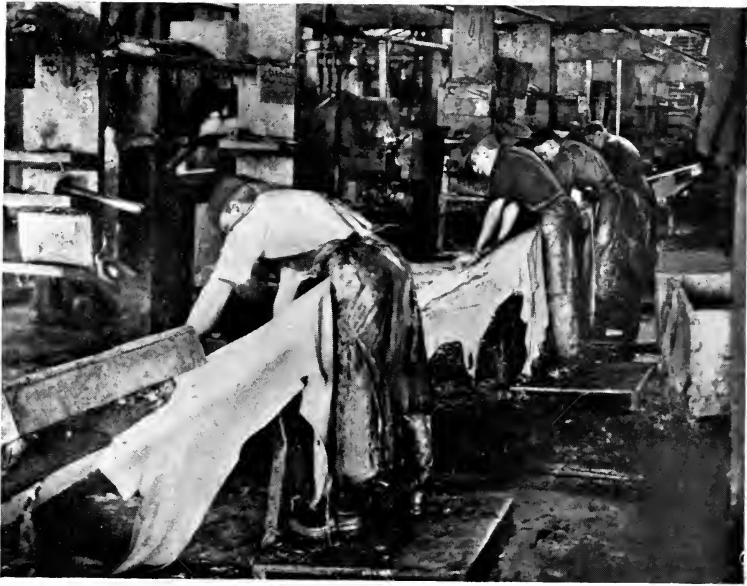
Trimming on the Beam
