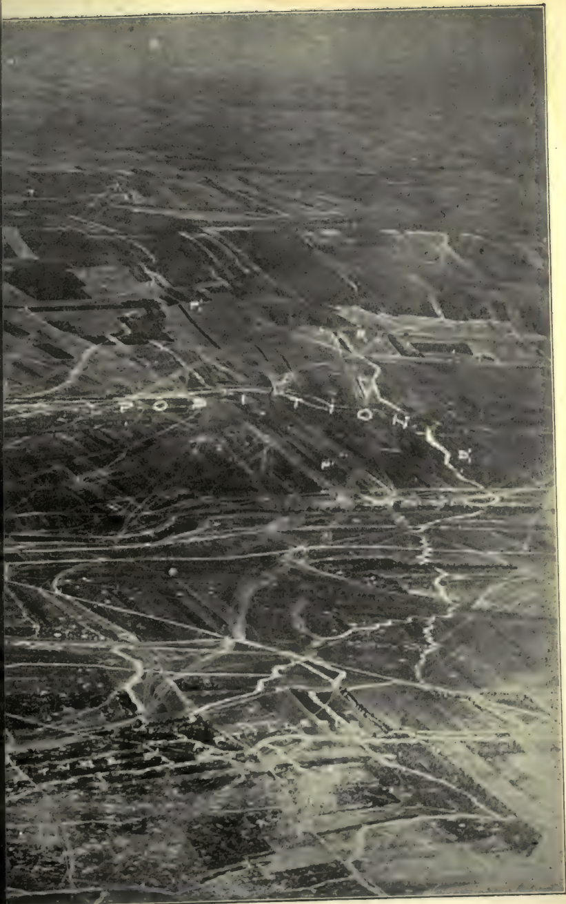
THE REAR OF THE TRENCHES
