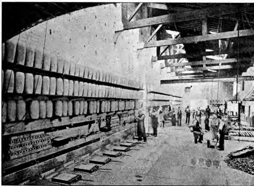
FIG. 40. The furnaces (tops at the floor level) and the crucible pits.
