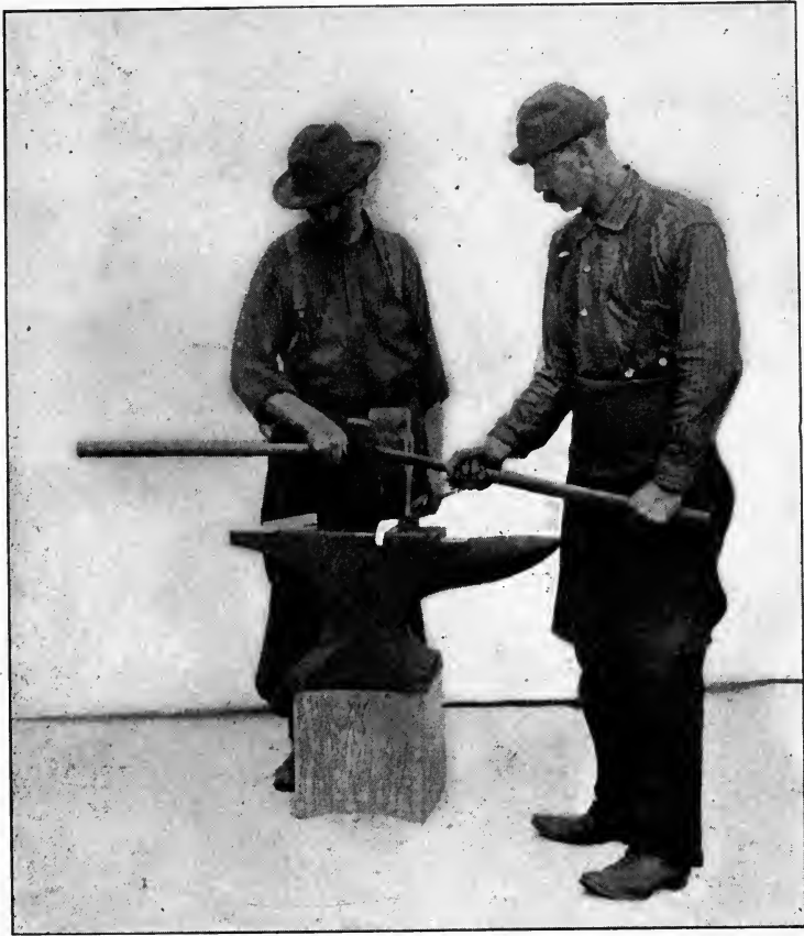
FIG. 52. Forming a bent side tool.
