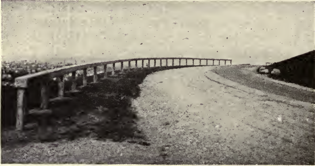
FIG. 44a.—Concrete Guard Rail.
