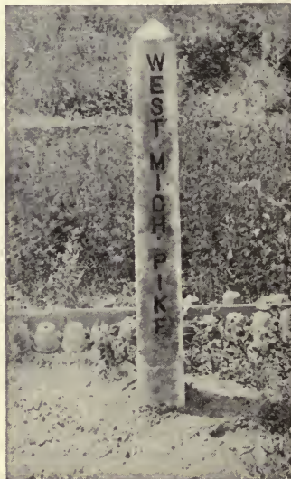
FIG. 177.—A Simple Concrete Road Marker.
