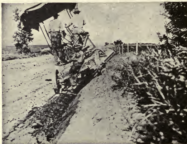
FIG. 77.—Trimming Off the Side with a Road Grader on a State-aid Project in Nebraska.
