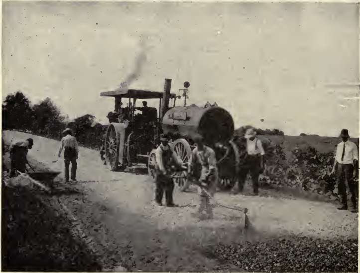
FIG. 164.—Constructing Bituminous Macadam Roads.
