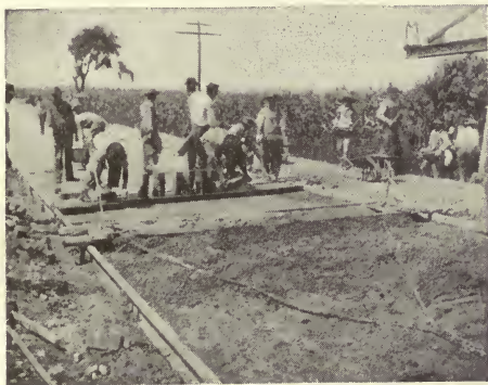
FIG. 126.—Laying Monolithic Brick Pavement.
