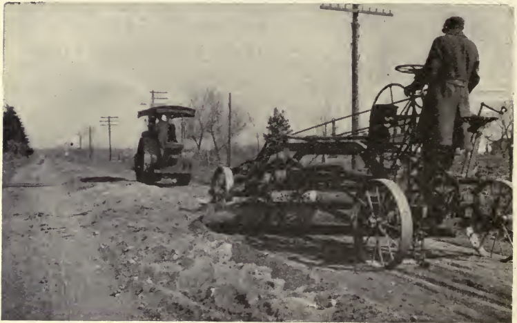
FIG. 99a.—Spreading Gravel with a Blade Scraper. Courtesy of Iowa State Highway Commission.
