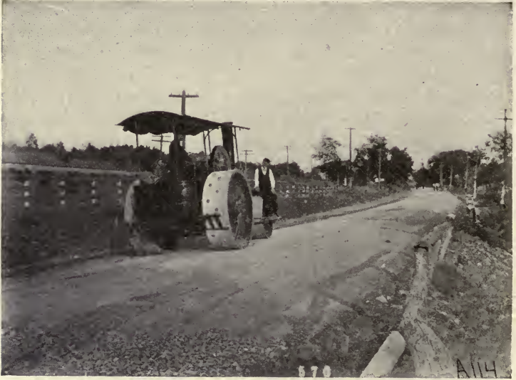
FIG. 109.—Rolling. Courtesy U. S. Dept. of Agri.
