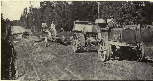
FIG. 76.—A Good Example of Grading Operations in Grant Parish, Louisiana.
