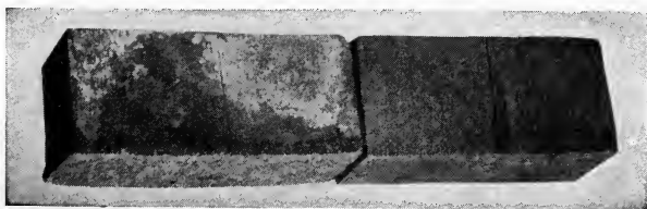
FIG. 128.—Showing Wear of Wood Blocks.
