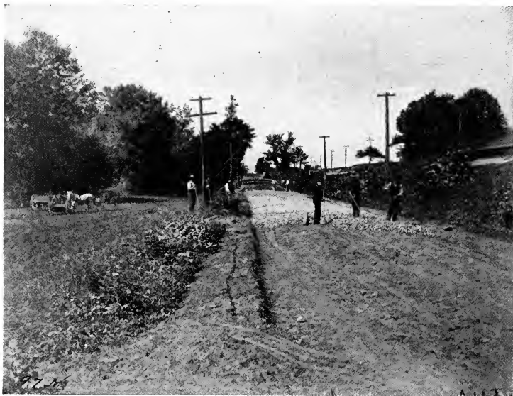
FIG. 108.—Placing the Stone. Courtesy U. S. Dept. of Agri.
