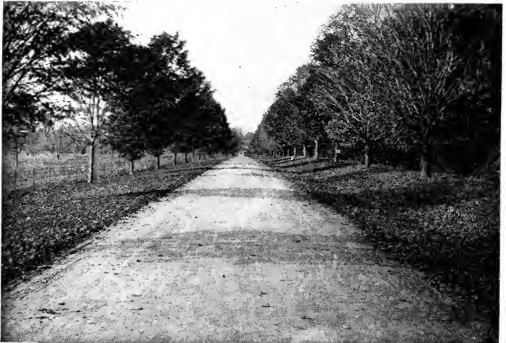
FIG. 110.—Finished Road. Courtesy U. S. Dept. of Agri.
