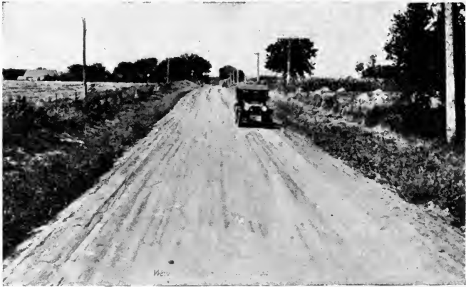
Fig. 91.—A Well-dragged Earth Road.
