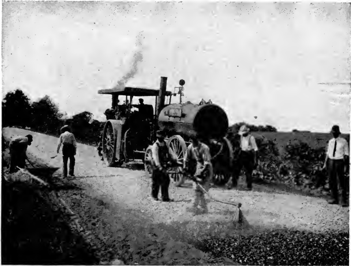
FIG. 164.—Constructing Bituminous Macadam Roads.
