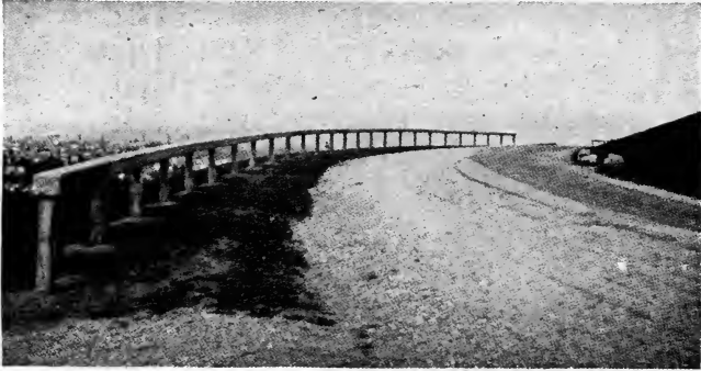
FIG. 44a.—Concrete Guard Rail.
