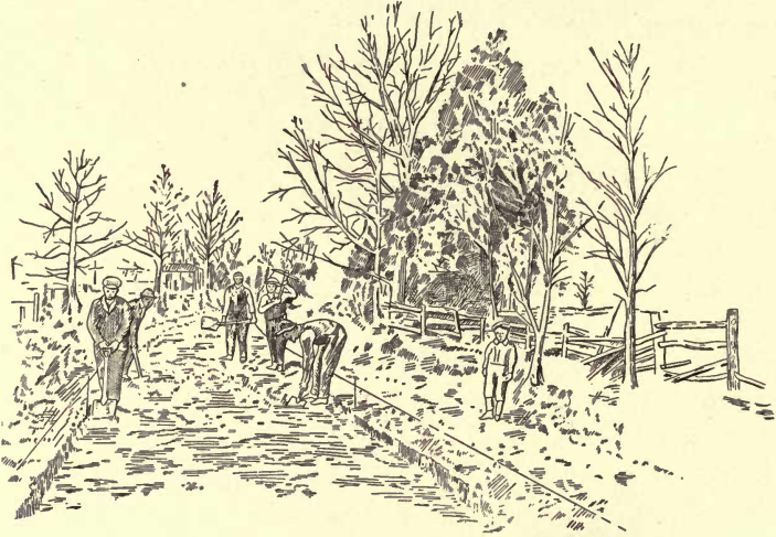
FIG. 42.—Excavating and Preparing Roadbed for Macadam Surface. Trench Construction.
