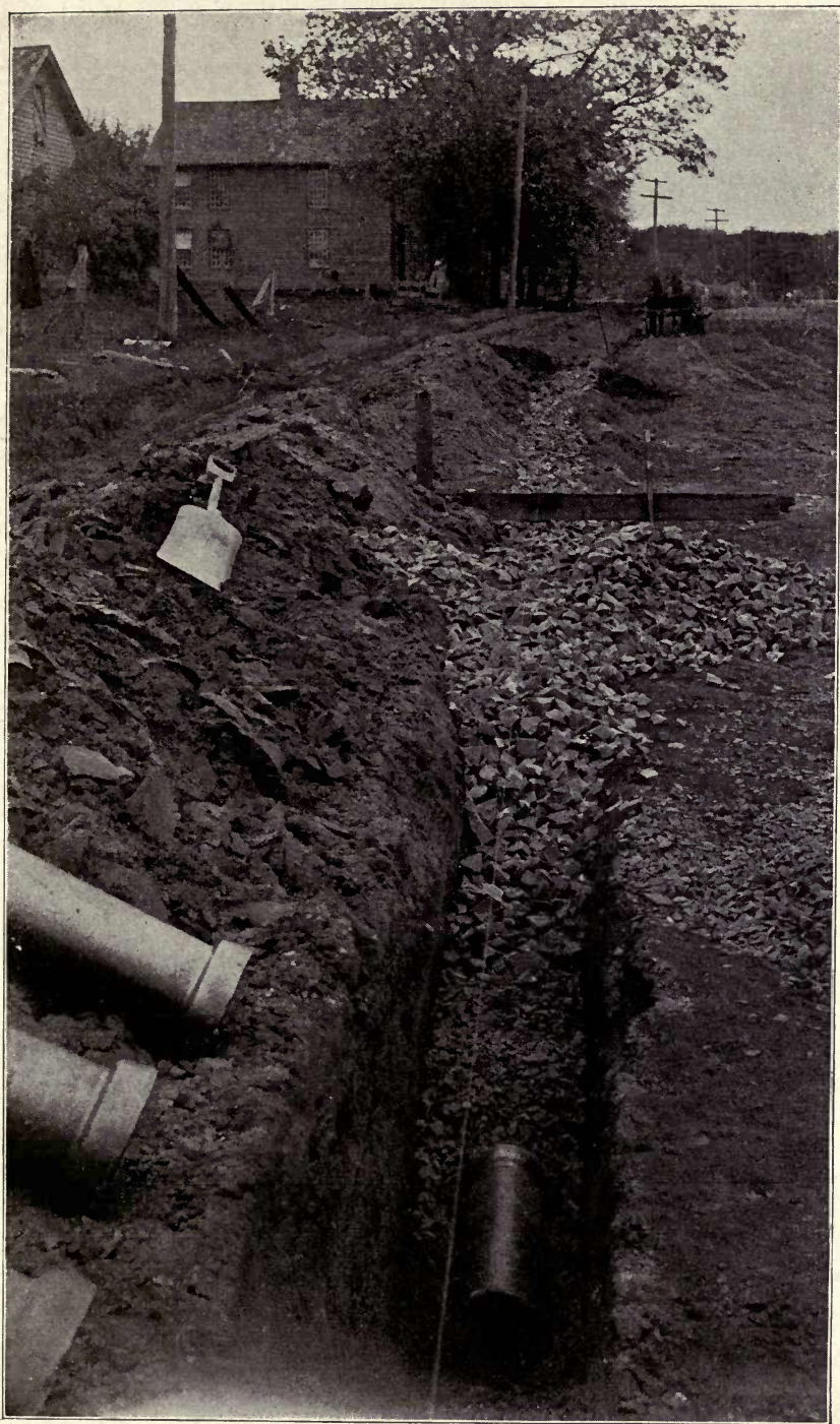
FIG. 18.—Detail of Drain.
