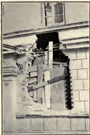
Military Academy, Belgrade, after the entrance of a 4-inch shell.
