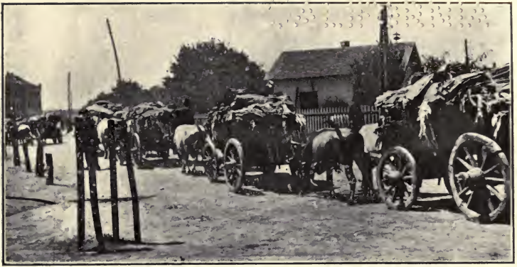
Transporting hospital garments which have been fumigated and "deloused."
