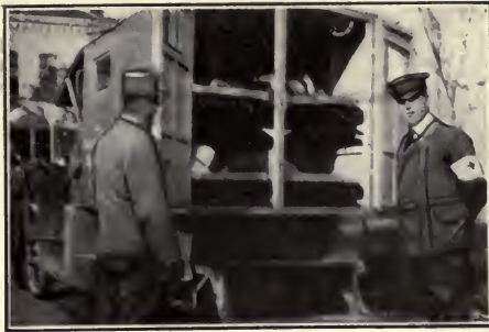
Austrian ambulance, also used by the Germans. High-powered, speedy, comfortable, and roomy. Equipped with a trailer, which makes it possible to carry 16 men sitting and 8 recumbent. The highest type used in the great war. (Dr. Jolly standing at right.)
