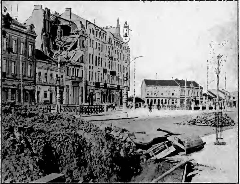
Grand Hotel Russia and principle square, Belgrade, after the bombardment, October 5, 1915. The finest hotel in all Serbia, and compares very favorably with our best hotels. It is practically all destroyed, especially the interior; all windows are broken. The large hole in foreground, made through the pavement by a 30.5, is about 16 feet deep and 30 in diameter. This has been a tragic square in the history of Belgrade. Here the "Committadji" were hung, and a civilian, until the Americans intervened and had them cut down. Here also a great many civilians were killed during the summer. As they were taking their afternoon stroll they fell victims to bombs dropped from hostile aëroplanes. The entire main street was torn up, as you can see in the photograph.
