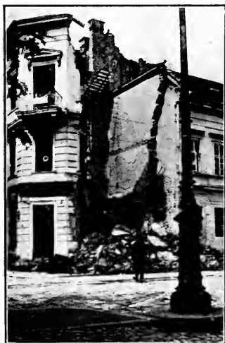
This was formerly a drug-store in the center of Belgrade. A large 42-centimeter shell passed entirely through the basement and the three stories down into the basement and exploded, completely demolishing the entire building, killing instantly several of its occupants and shattering windows for squares in the vicinity.
