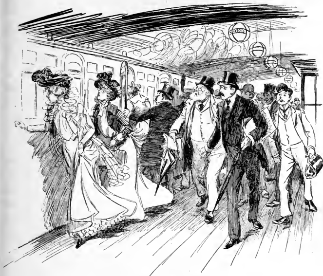
An Underground Station.
