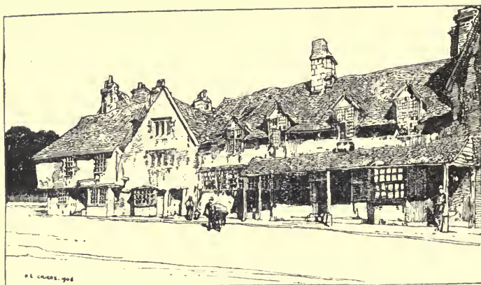
Faringdon. Part of Church Street, now demolished.
