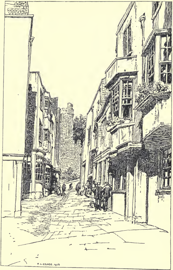
Windsor, Market Street.
