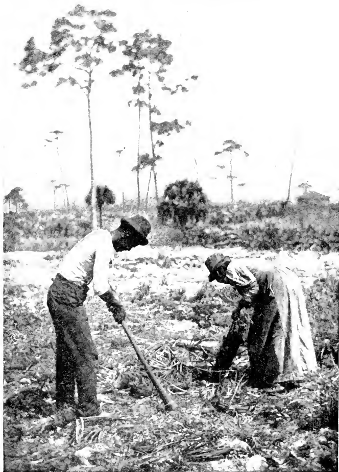
GRUBBING UP PALMETTO SCRUB
