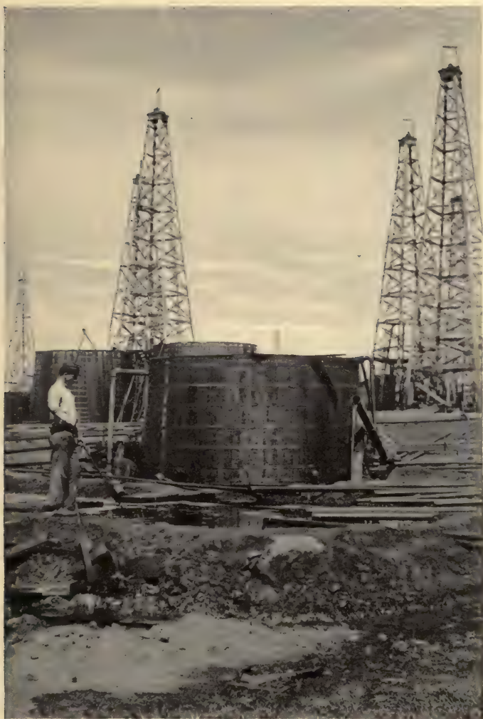
Some of the tanks among the derricks
