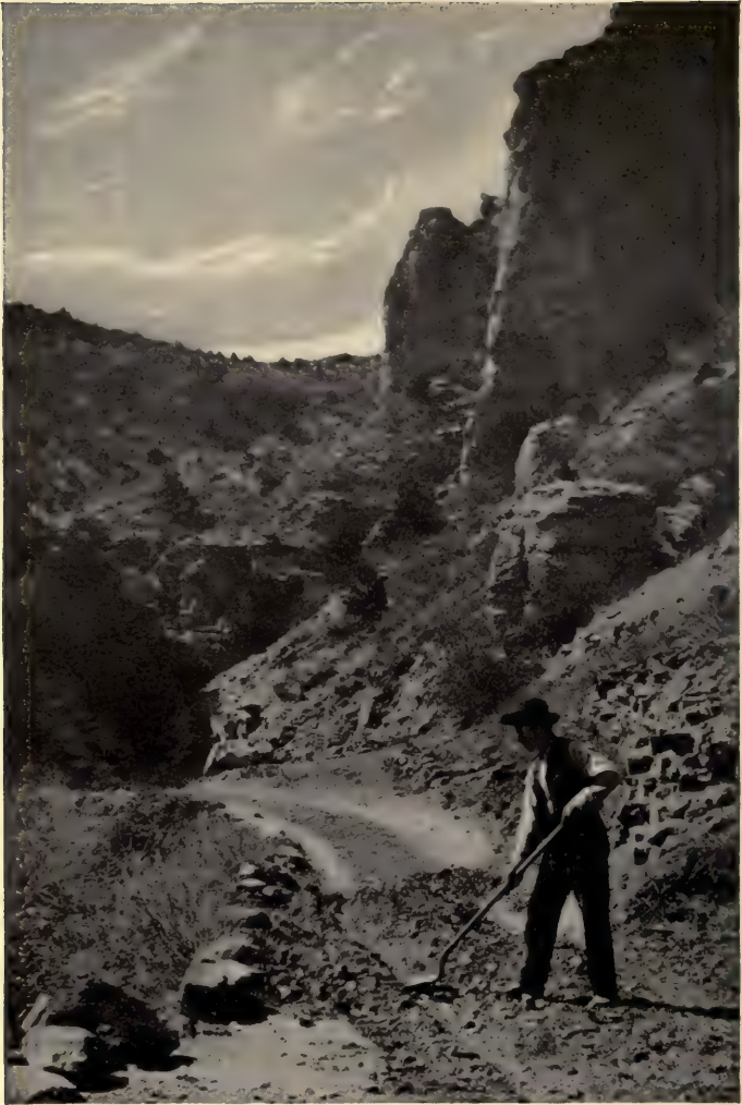
Working on the road
