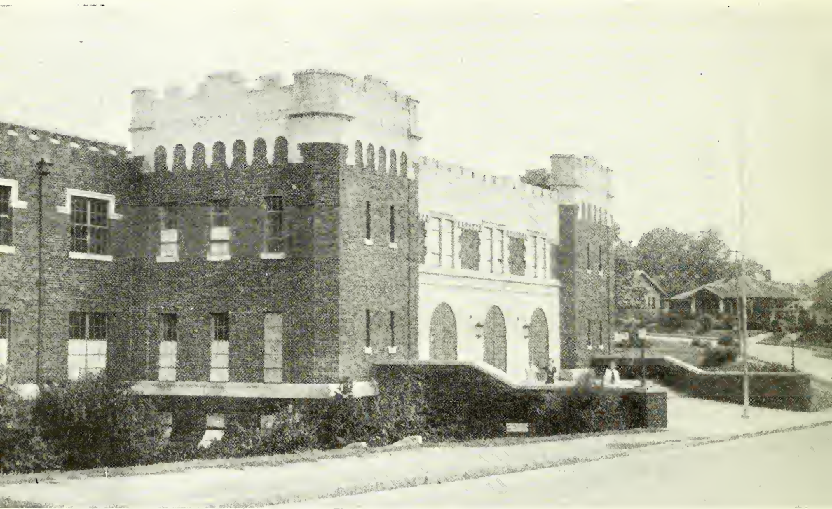
City Armory-Auditorium, Charlotte
