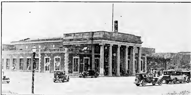
Southern Railway Passenger Station.
