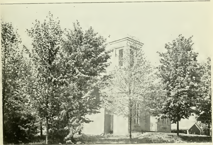
THE HIRAM CHURCH: ERECTED IN 1856; BURNED MAY 25, 1897.
