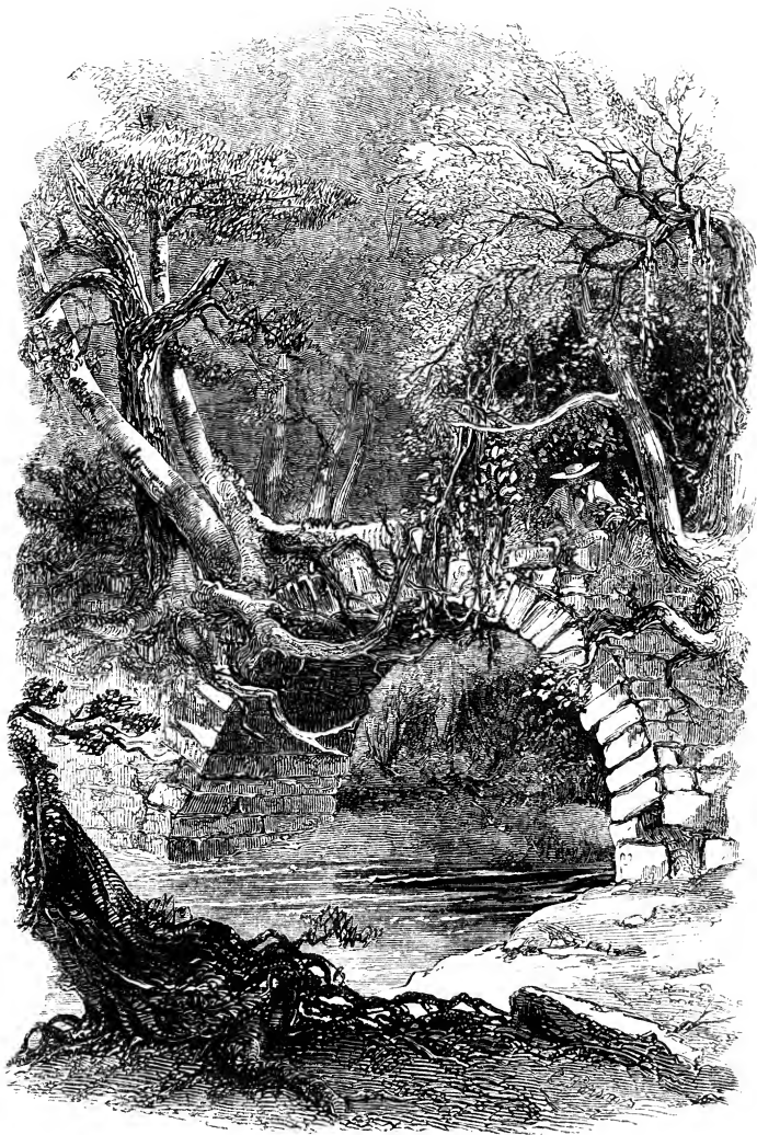
ANCIENT BRIDGE AT OLD PANAMA.
