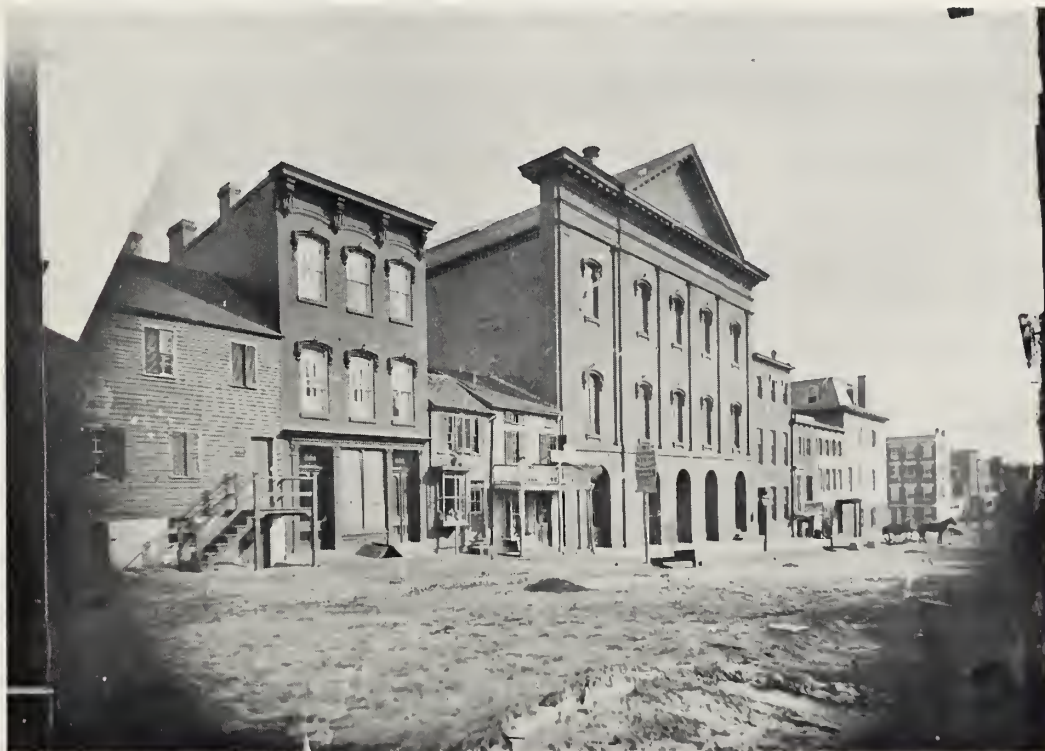
Ford's Theater building about 1870. The changes made to the west front and the roof in 1865 when the theater was converted into an office building can be seen by comparing this photograph with the earlier one. (Reproduced from a photograph by an unknown photographer in the Lincoln Museum collection.)
