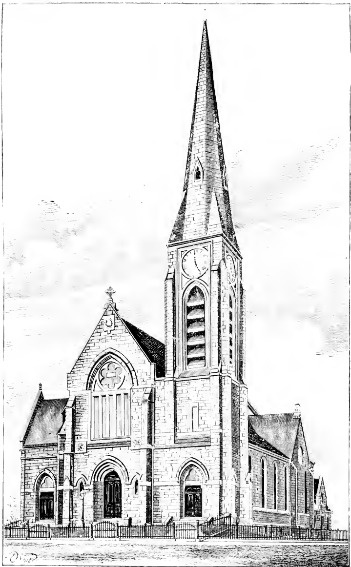
FIFTH MEETING HOUSE—ERECTED 1877-78.
