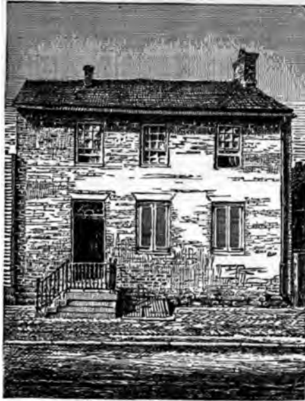
Davison Fillson, Photo.
