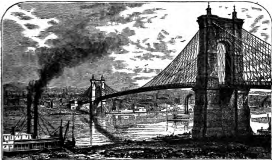
THE SUSPENSION BRIDGE.
