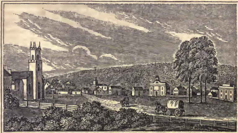
View of the Public Buildings at Angelica.
