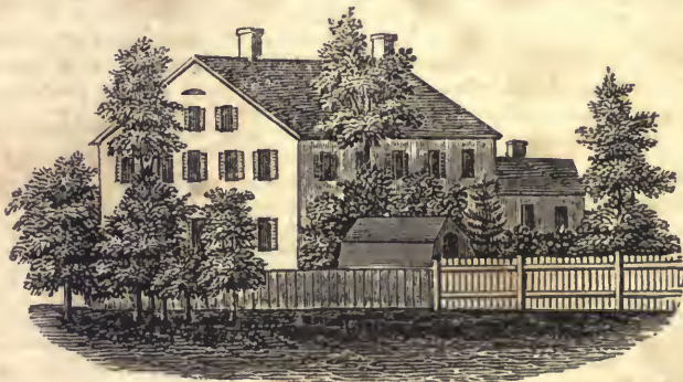
South view of the Jemima Wilkinson house.
