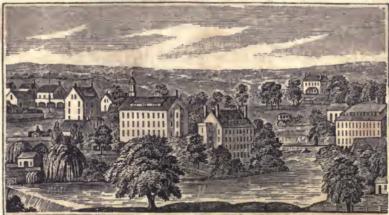
Factory Buildings in Matteawan, Fishkill.
