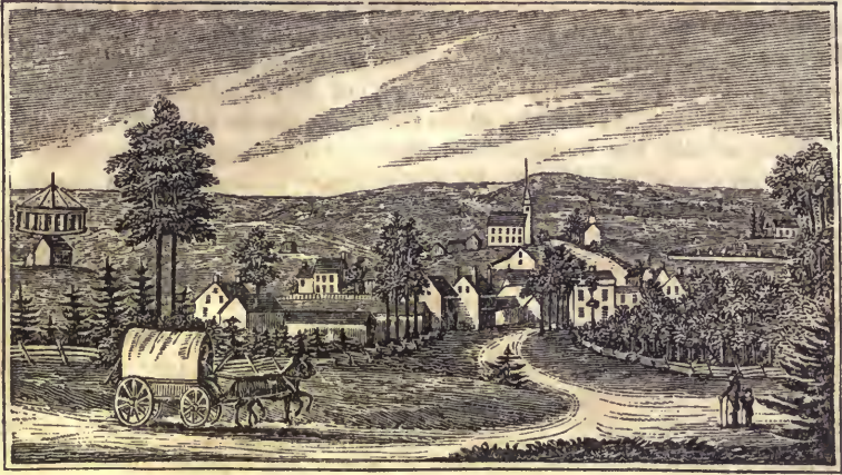
Western view of Huntington Village.
