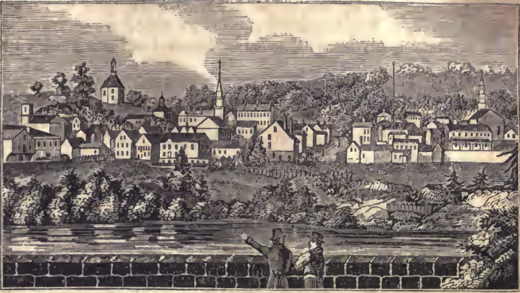
Southern view of part of the Village of Little Falls.
