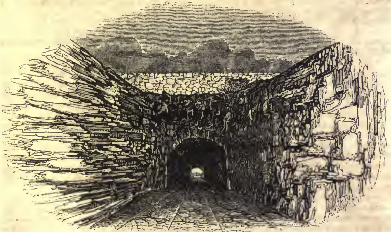
Northern view of Harlem Tunnel.
