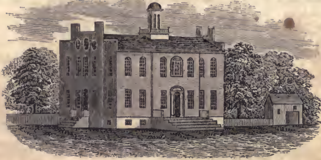
South view of the courthouse in Waterloo.
