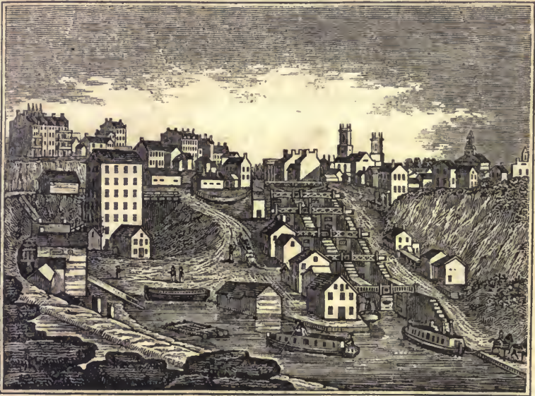
Northeastern view of the locks at Lockport.
