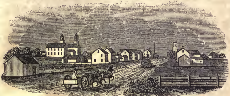
Western entrance into Monticello.
