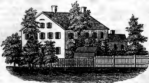
South view of the Jemima Wilkinson house.
