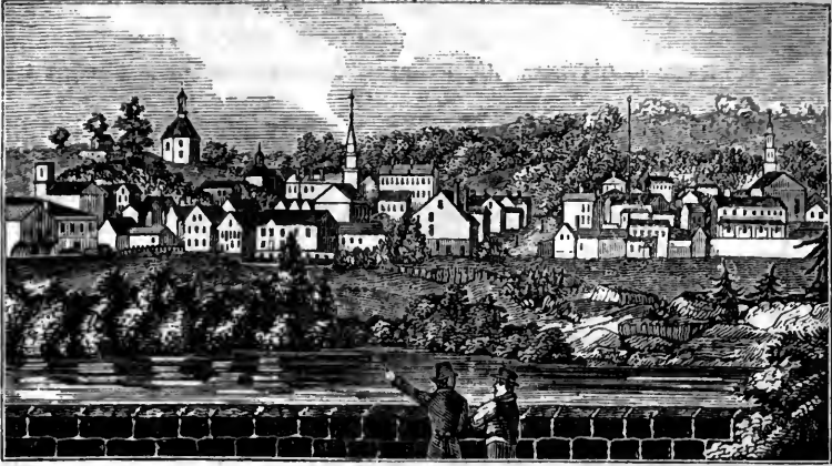
Southern view of part of the Village of Little Falls.
