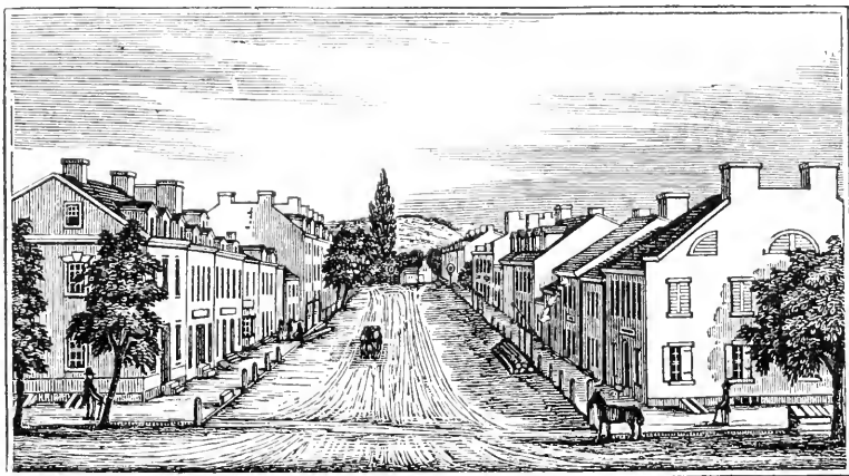
View in the central part of Lewistown.
