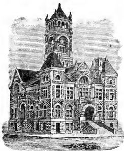
THE PERRY COUNTY COURT-HOUSE, NEW LEXINGTON.
